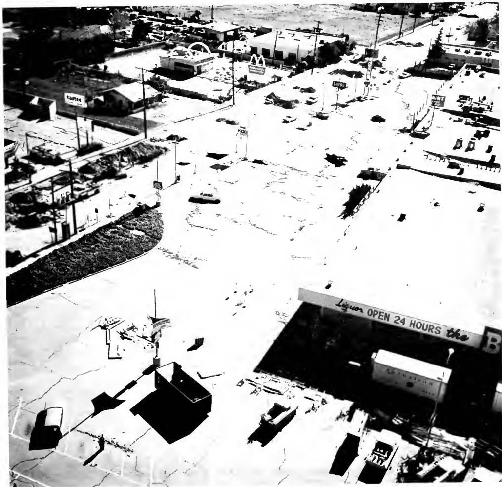
Photo 6. The commercial area at the southwest corner of Glenoaks Boulevard and Hubbard Street was damaged by displacement, lurching, and strong ground motion. Photo courtesy of Robert E. Wallace, U. S. Geological Survey.
